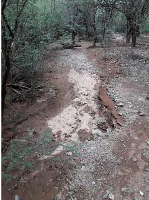
Figure G1-21. 1,700 m. Depression (1 m wide by 3 m long by 20 cm deep), created by rain water flow
